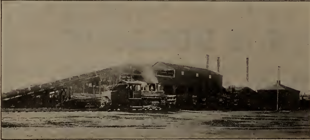
COLLIERIES AT WESTVILLE, NOVA SCOTIA.
